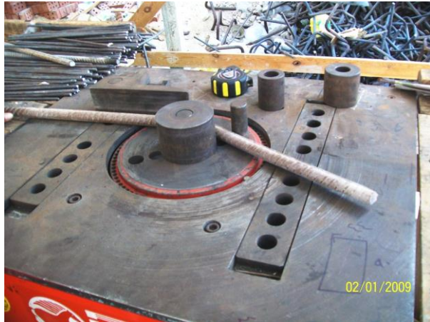
Fig. 10. Bending machine for steel bars during construction.
