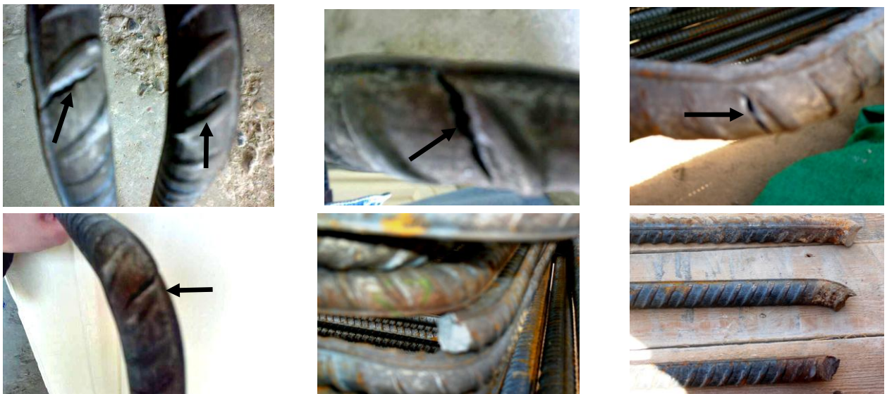
Fig. 13. Serious cracks and fracture of steel bars with different diameters on site [provider 'Z'].
