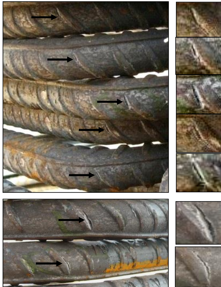
Fig. 12. Cracks appeared in most of the 22 mm- steel bars from provider 'Z' on site.
