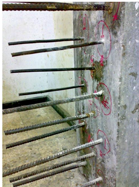
Fig. 23. Testing of concrete column prototype.
