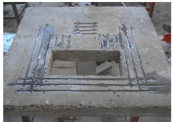
Fig. 10. Installing NSM FRP reinforcement in the slab.
