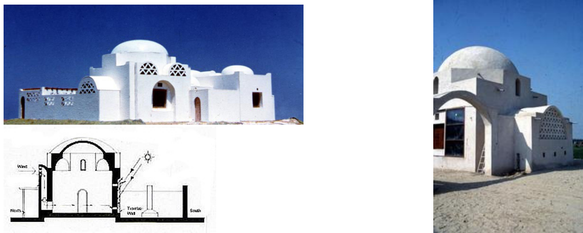
Fig. 4. Maxi project: a private residence in South Tahrir designed by Samir Bayoumi ,1987. Cross-ventilation, wind tunnels humidifying the air, Trombe walls and the planted patio constitute the main passive cooling systems, while direct and indirect heat gain through glazed windows and Trombe walls are used for passive heating [9].
