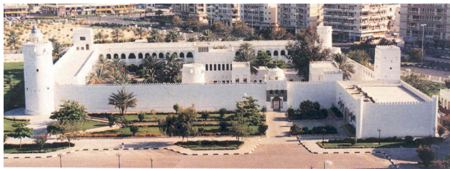
Fig. 2-a. Square enclosure with two diagonally placed towers (Qasr Al-Husn in Abu Dhabi).
