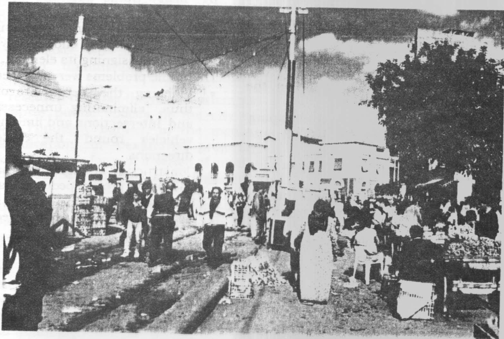
Fig. 2. Midan Misr Station (during upgrading).
