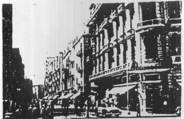
Figure 3.2.8. Metropol Hotel, Alexandria Source Ibid.
