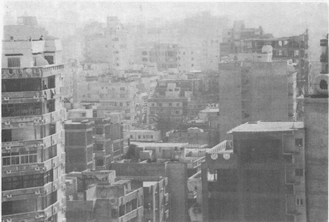
Figure 2. Disorder and poor treatment of elevations.
