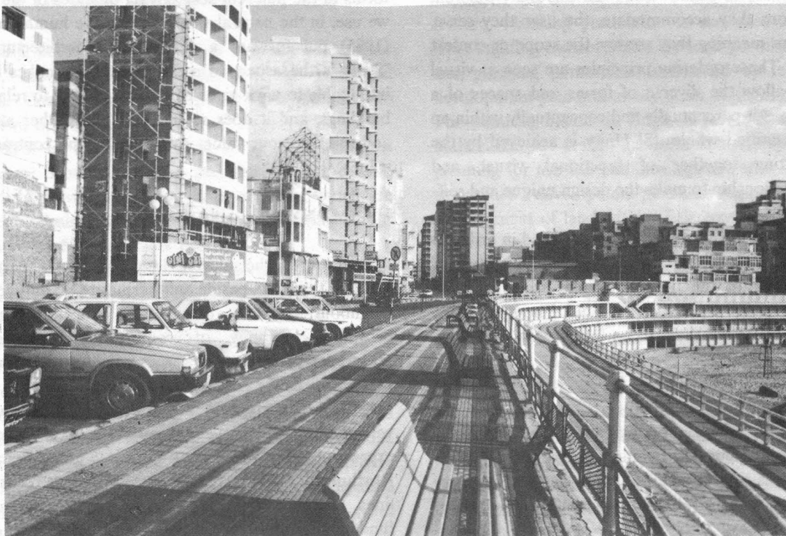
Figure 5. The absence of Landscape treatment and features.
